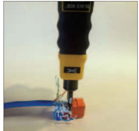
Cable being punched down.
