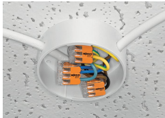
Lighting distribution in a ceiling canopy
