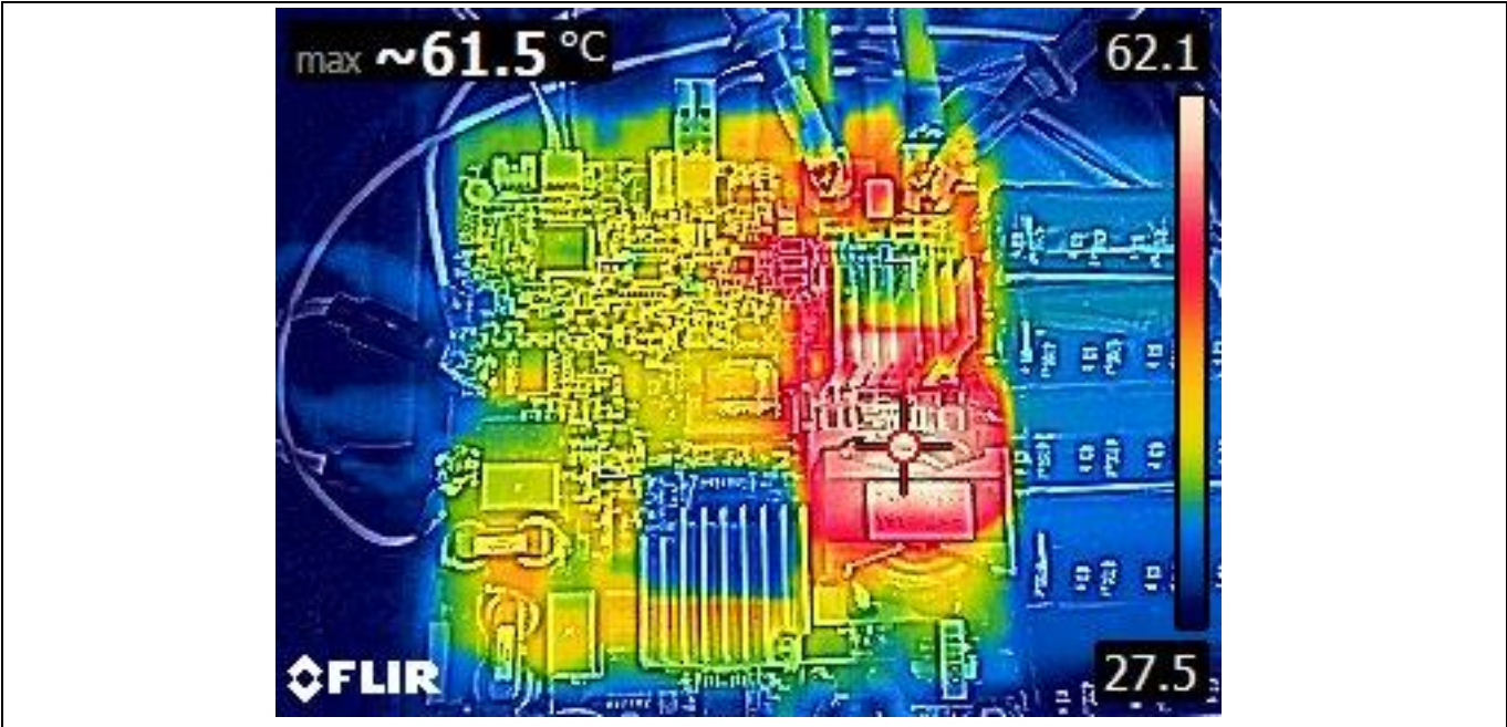
Figure 131 REF_500W_CYCLO_BDSGAN thermal image
