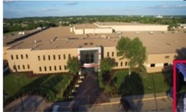
Lincoln, Nebraska Sending Plant
