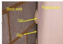
Drylined walls will generally sound "hollow" when you tap them. At certain points they will sound dead. This is a point where the builder has used some adhesive cement to stick the plasterboard to the wall. These walls are a challenge for conventional fixings, as there is an awkward, irregular gap between the plaster and the wall.
