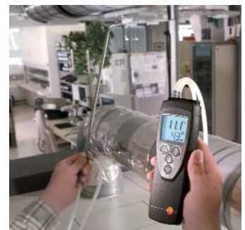
Measuring process air
